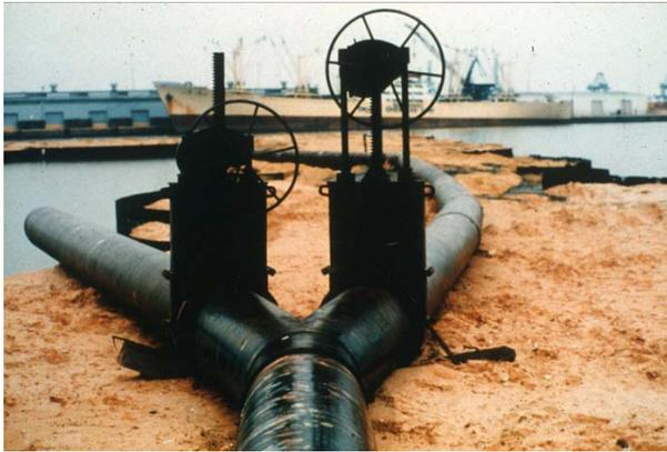
Figure 2. Y-valves on the pipeline separated the clean and contaminated sediments during disposal operations.
