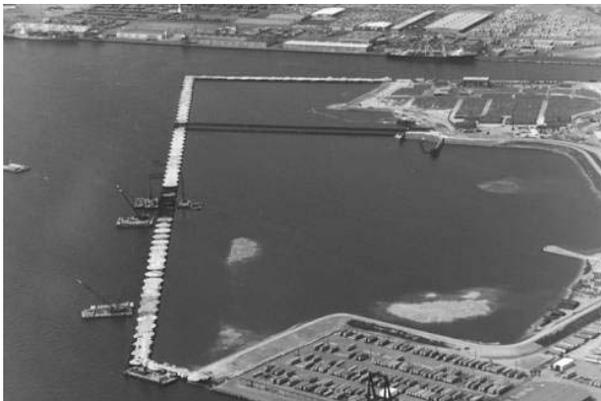
Figure 3. Seagirt nearshore CDF during construction.
