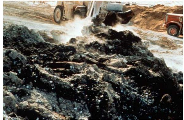
Figure 7. Odor neutralizing foam sprayed on sediment stockpiles.
