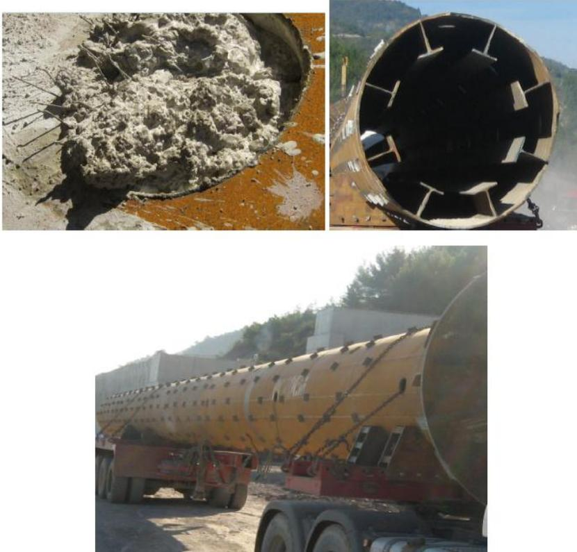
Figure 6. View of a CFT Pile
