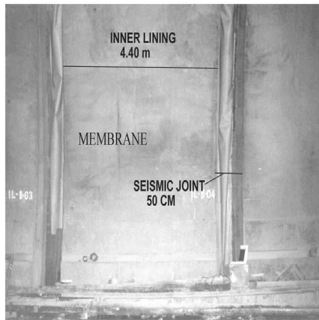
Figure 6. Seismic joints of 4.40 m spacing and 0.50 m spanning are currently being constructed at the Bakacak Fault crossing.
